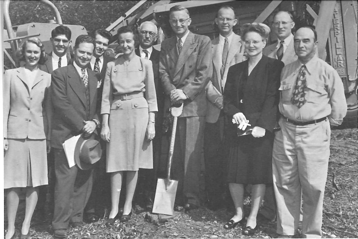
Ground breaking of the men's residence area. (From left) AWS President Marillyn McCormick; AMS President Henry Culbertson; contractor Paul Spencer '28; ASOC President Robert Finch; Comptroller Janet Hoit '27, then manager of residence; architect Myron Hunt; President Coons; Dean of Men Benjamin H. Culley; Las Amigas Mothers' Club President Mrs. Leslie L. Penn; Superintendent of Maintenance Harold Hare; Superintendent of Grounds Frank Collier.
